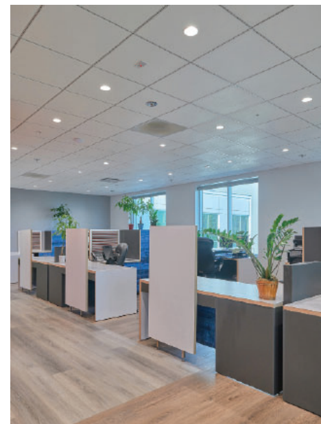
Figure 3. The facility includes Title 24-2019 compliant control plans for open and private offices, conference rooms, restrooms and training rooms.
